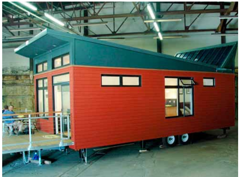
The PowerPod is a 500 square foot modular green building with an active solar array, remote building monitoring system, high efficiency lighting and water use, heavy insulation and airtight exterior, radiant floor heating, solar windows, rainwater collection scupper, and optional composting septic and grey water technology. The Yellow Barn Music School in Putney, Vermont is using eight PowerPods for its music lessons. www.yellowbarn.org
