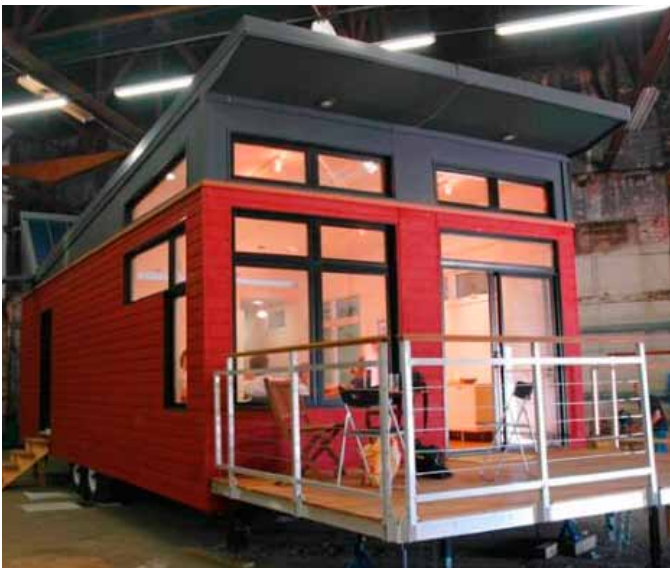
The PowerPod is a 500 square foot modular green building with an active solar array, remote building monitoring system, high efficiency lighting and water use, heavy insulation and airtight exterior, radiant floor heating, solar windows, rainwater collection scupper, and optional composting septic and grey water technology. The Yellow Barn Music School in Putney, Vermont is using eight PowerPods for its music lessons. www.yellowbarn.org
